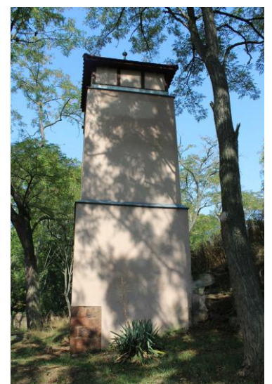
Trafohaus in Gimritz
